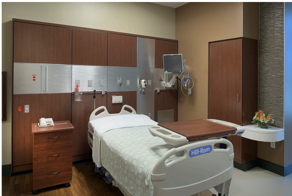
Premanufactured ICU headwall from Hill-Rom, Texas Health Hospital, Carrollton TX
